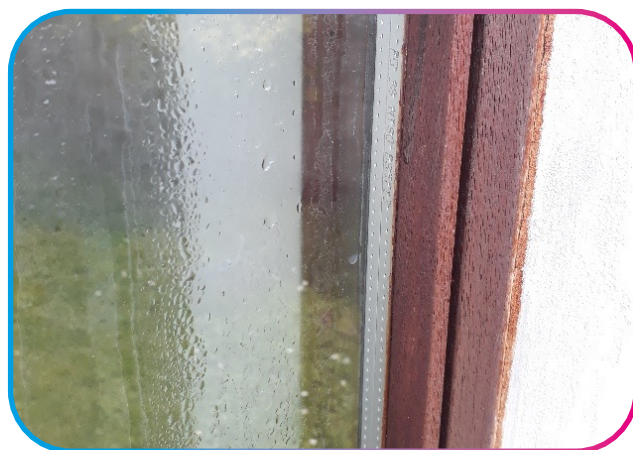
This old wooden window has 12mm glazing that has 'blown' (got condensation between the panes). It needs major maintenance - better to replace?
