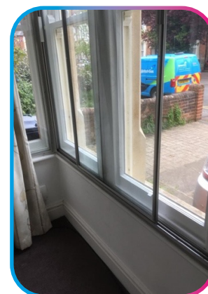
Secondary glazing on sash windows.
