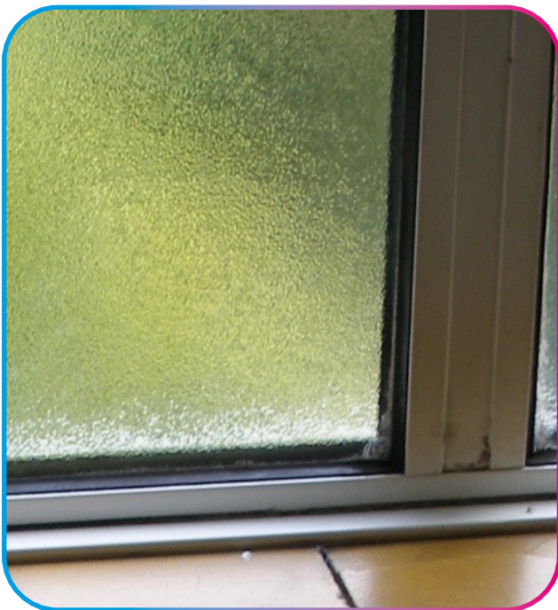
Old style, old technology, probably worth replacing even if not in need of maintenance, especially if there is condensation on the frame in winter.
