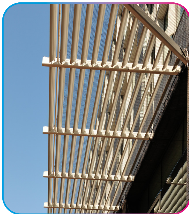
External shading 'Brise Soleil' to reduce overheating of a commercial building.
