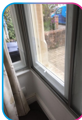
Secondary glazing on sash windows.
