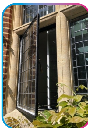
Secondary glazing in a listed building
